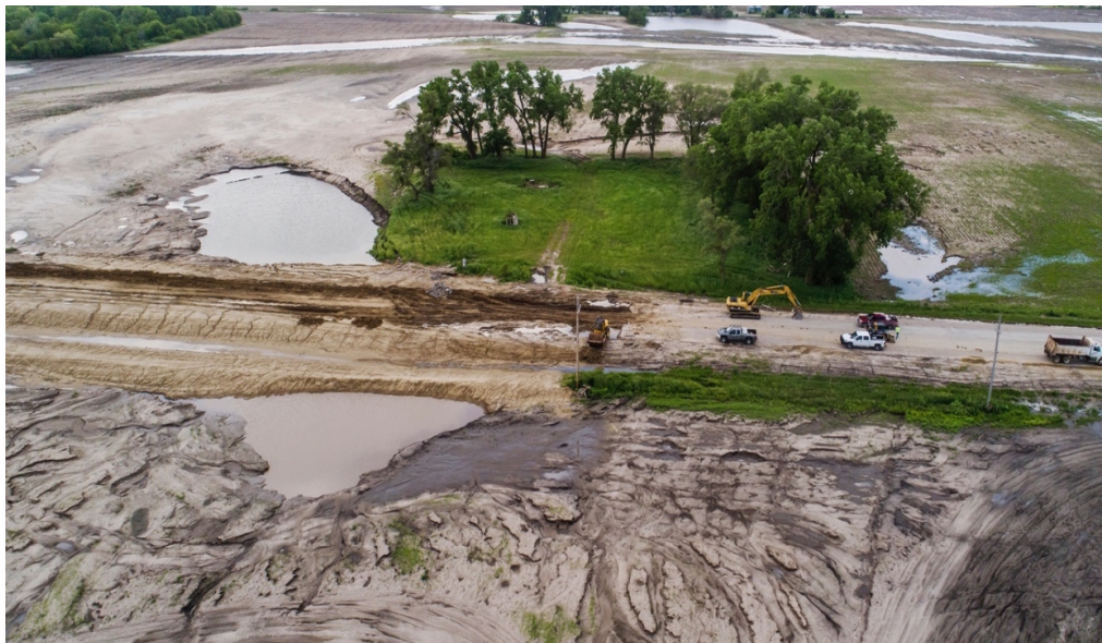
Figure 10 – Photo of Washed Out Road Under Repair
